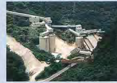
選鉱 Crushing and screening
