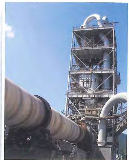
プレヒータとキルン New suspension pre-heater and Rotary kiln
